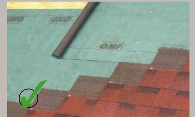
Tear off the old shingles and start building up with OSB, Underlayment and Cambridge Xtreme 9,5°.
